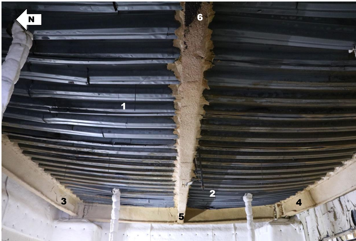
Fig. 36. Post-test photograph of the floor specimen soffit.
